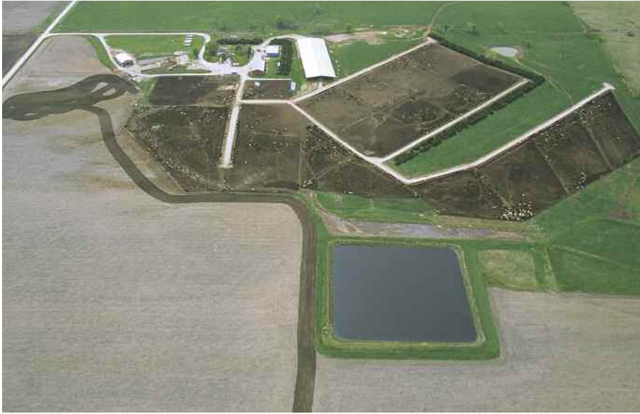
A Kansas feedlot operation with waste management lagoon in the foreground.
